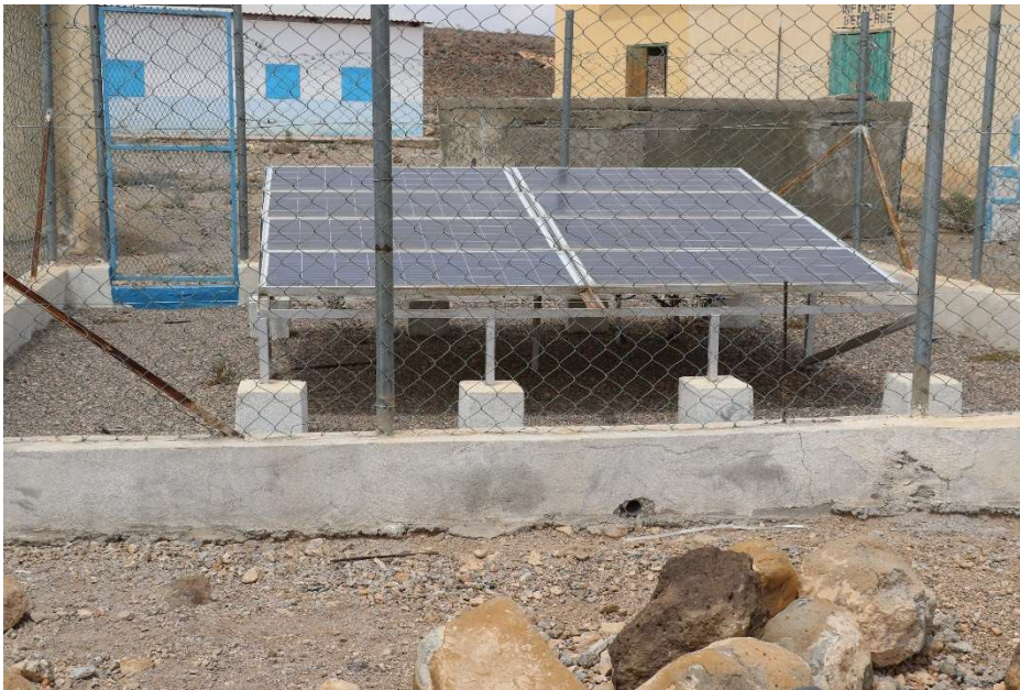
1 A PHOTOVOLTAIC PANEL OF A SOLAR POWERED WATER SUPPLY SYSTEM IN BEYADEH
