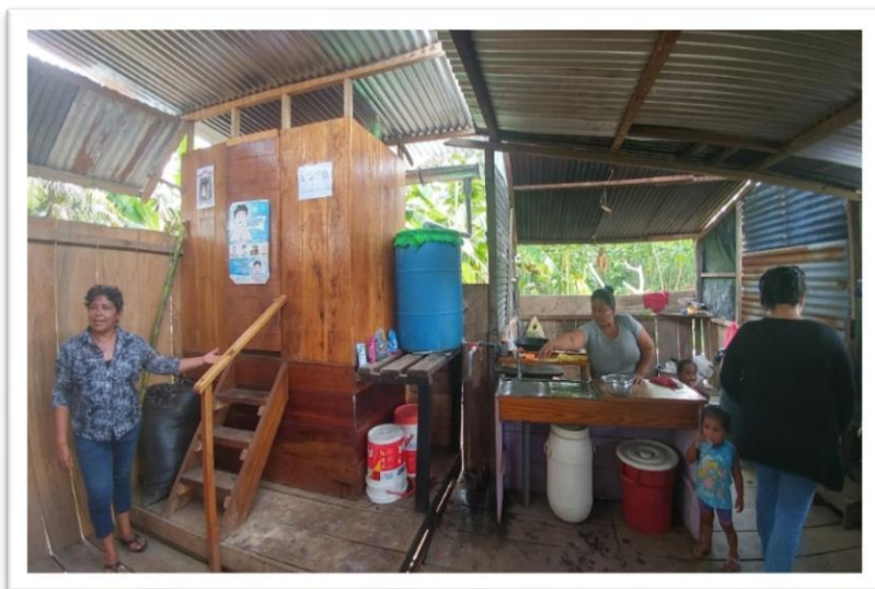
Picture 1. Rainwater collection system, accompanied by a composting dry ecological toilet in the CCPP Manco Cápac.
