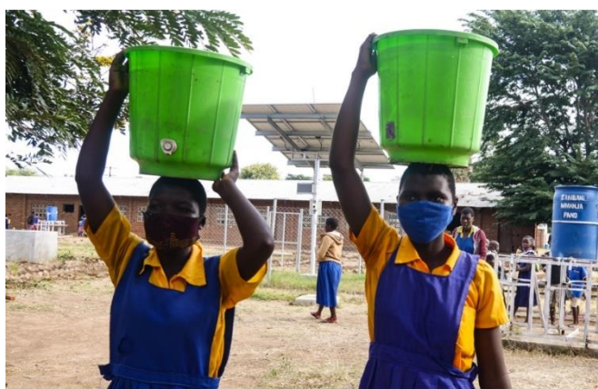
Girl learners carry water buckets as they walk past the newly installed solar water reticulated system, © UNICEF/UN0516077/Chagara
