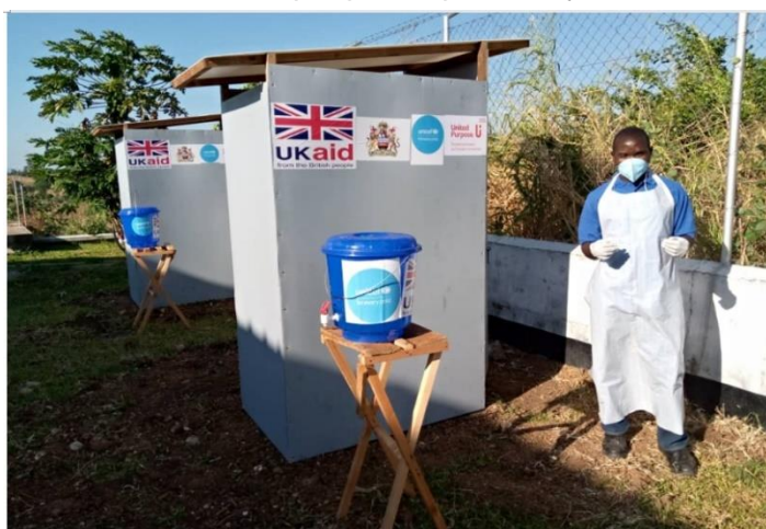
Latrines and handwashing buckets at the emergency treatment unit in Mchinji. They were installed with funding from UK Aid © United Purpose/2020/Chifundo Mandala
