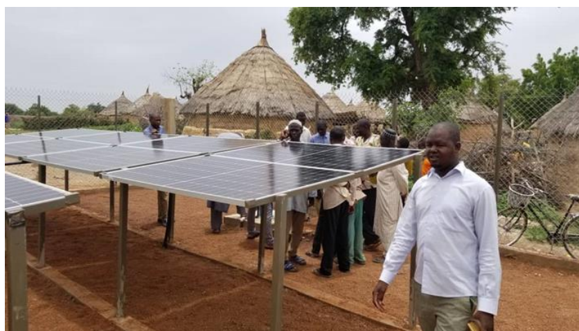
The rehabilitated and extended mini water supply network in Banteri village in Tillaberi region (DEMI-E, 2021)
