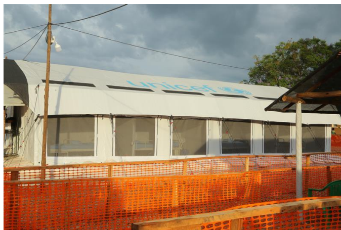
Figure 2: Ebola Treatment Unit in Mubende District that was constructed by MSF International with support from UNICEF and WHO. Credit: © UNICEF Uganda/2022/Stuart Tibaweswa
